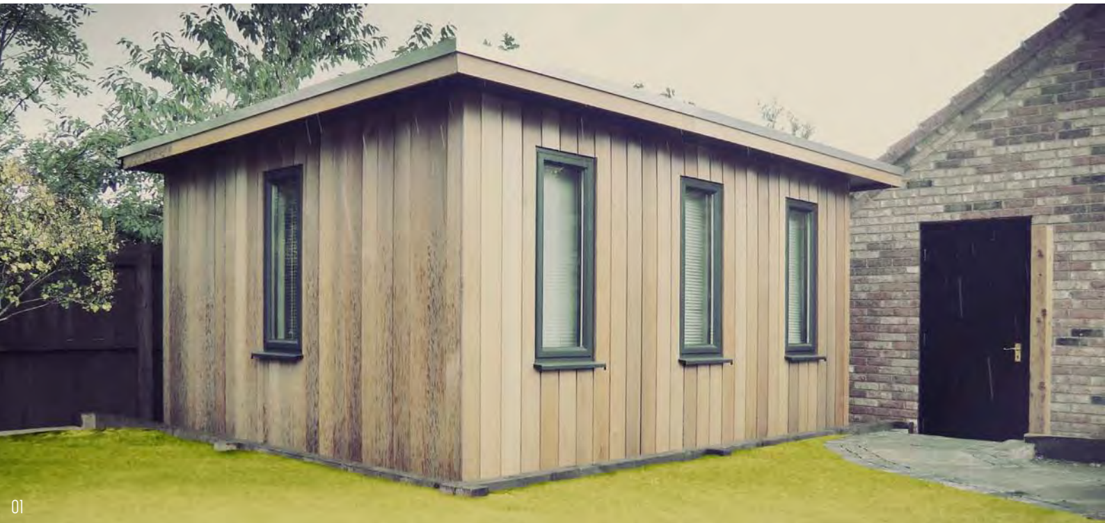
01 | Pod 3 with extra window installed in a sunken garden terrace to reduce it's height in the garden
